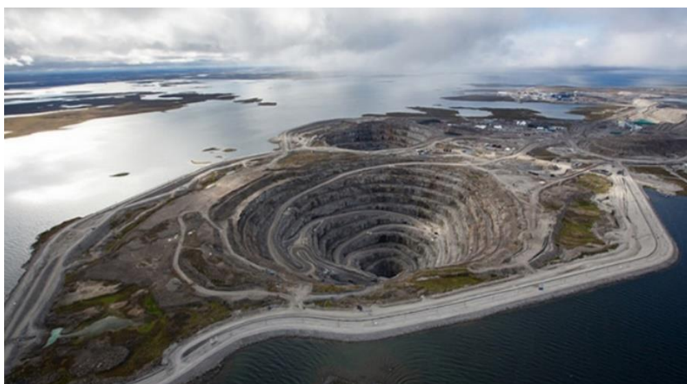
Diavik diamond mine summer A154 dike and open pit. To safely open-pit mine its ore bodies, extinct volcanoes located just offshore under the lake waters, dikes were built. Courtesy: Copyright © 2016 Rio Tinto.
